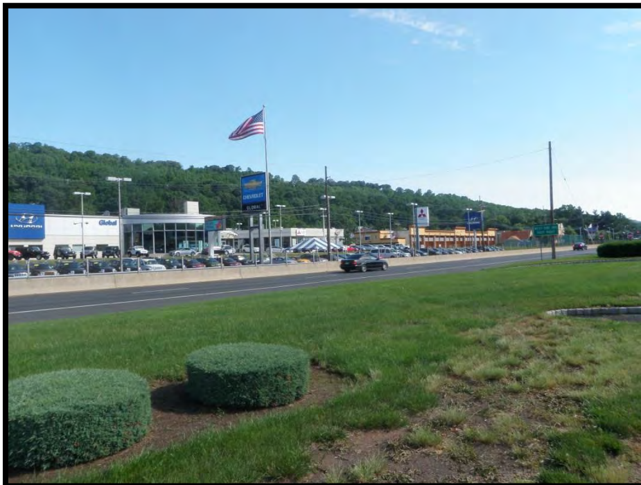
Photo B: View looking north of Route 22 showing northward increase in elevation associated with the base of the Watchung Mountains.
