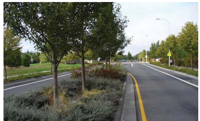
This vegetative median in Washington State helps to calm traffic and mitigate storm water runoff.
