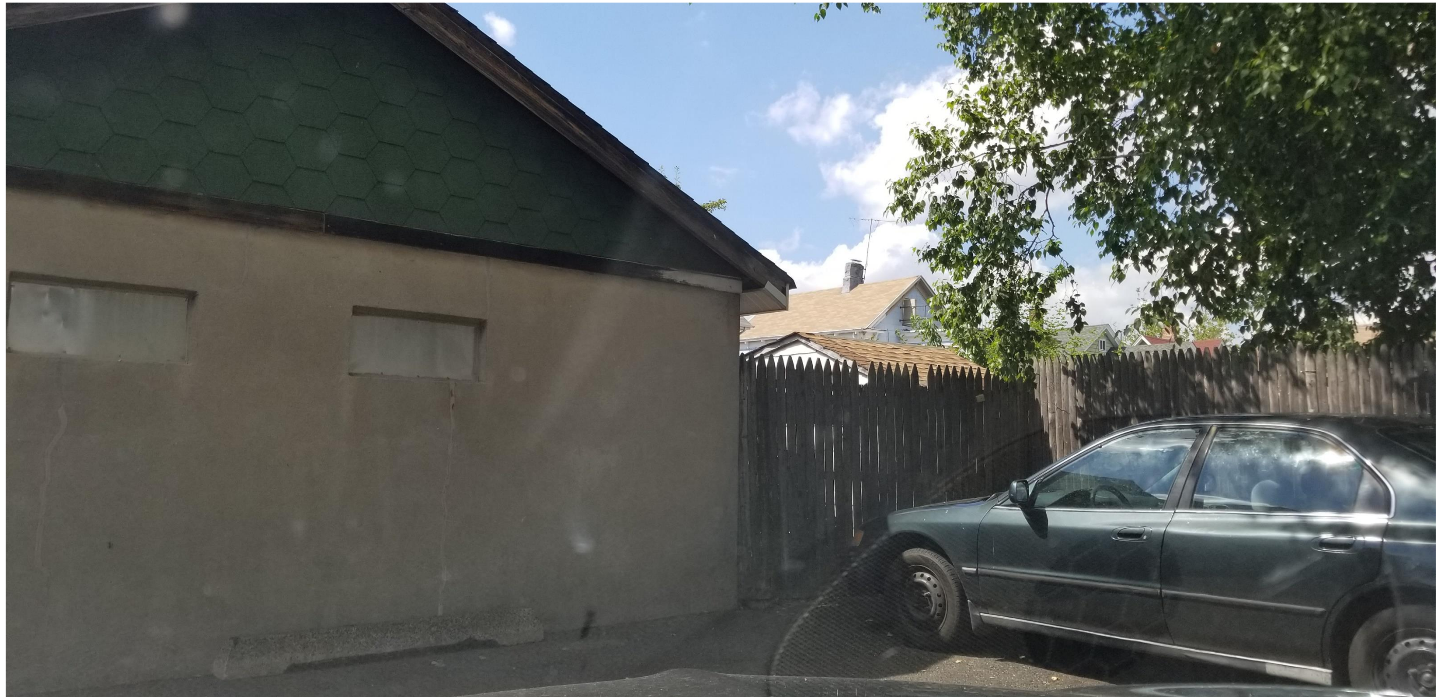
VIEW OF SUBJECT REAR PARKING AREA SCREENING AND ADJACENT MASONRY SHED (TAKEN BY JOHN MCDONOUGH JULY 29, 2020)
