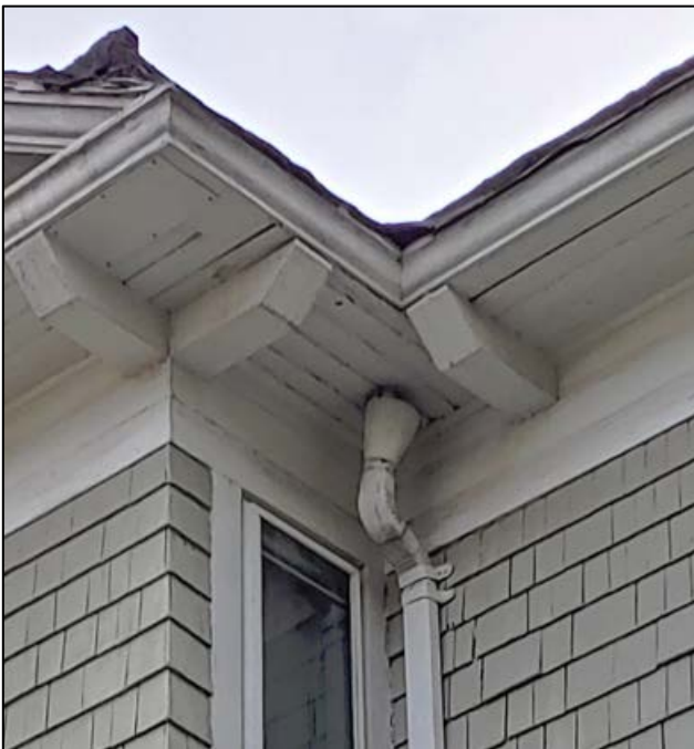
Appropriate downspout placement.
