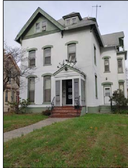
Satellite dishes installed on main entry.
