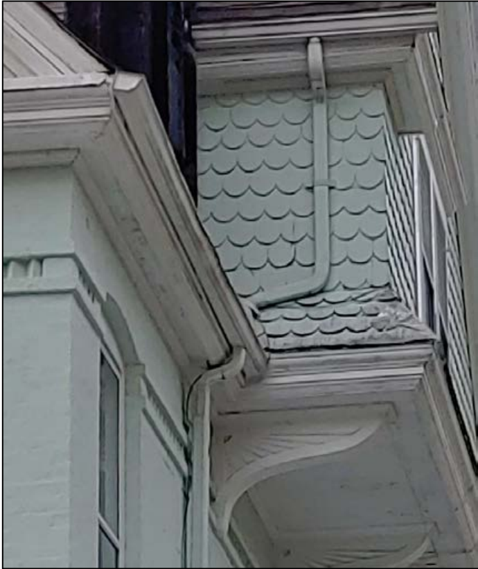
Appropriate downspout treatment.
