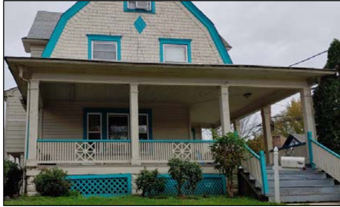
Appropriate porch ceiling, lattice, railing, and steps.
