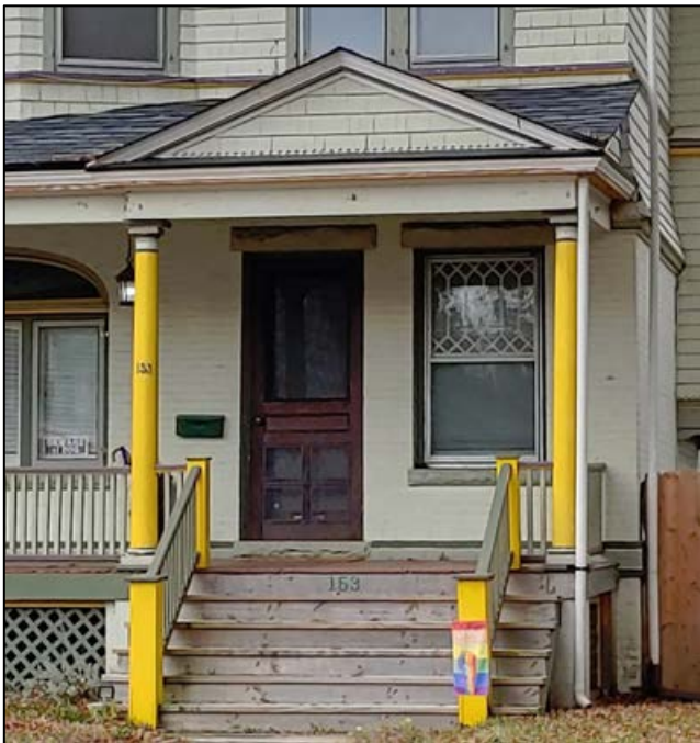
Appropriate wood railing.
