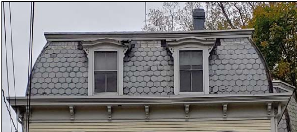
Convex mansard with slate shingles.
