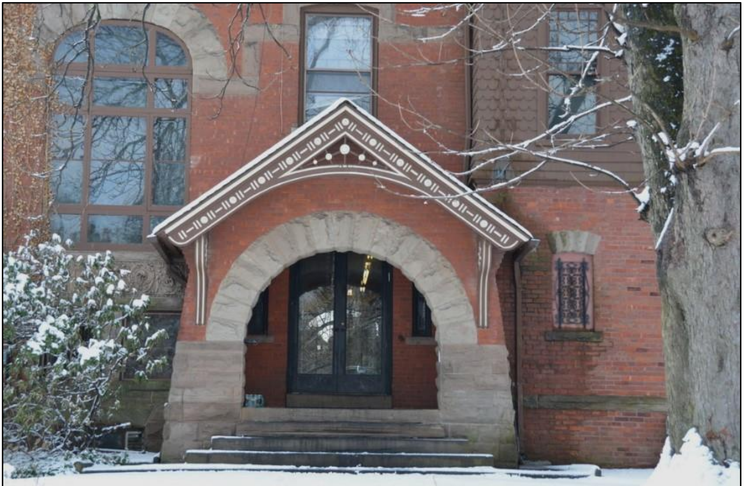
Brick and Masonry Facade 21 Rockview Avenue
