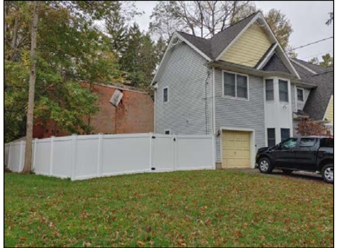
Inappropriate vinyl privacy fence.
