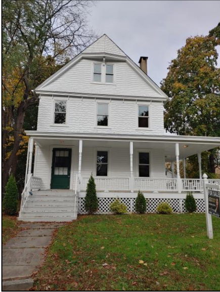
No street-visible air conditioning units.
