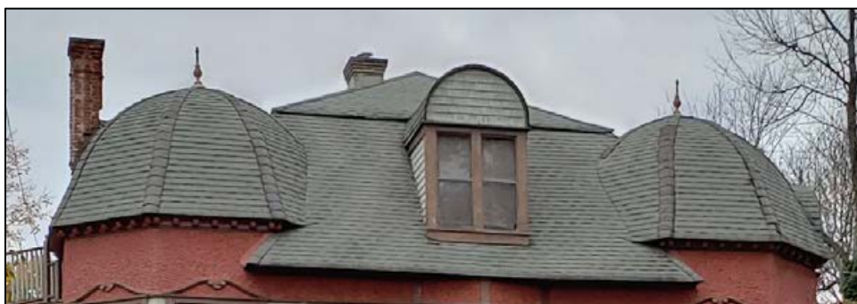
Asphalt shingle roof with towers and dormers.
