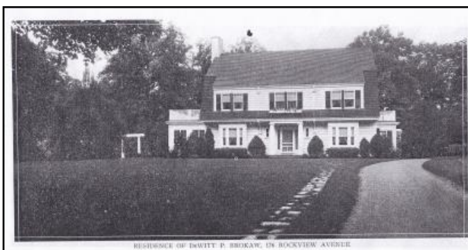
Figure 29 Ca. 1917 view of 176 Rockview Avenue Published in the Plainfield Courier News Showing Modern Landscape and Public Safety features (e.g. sidewalks, crosswalks, etc...).
