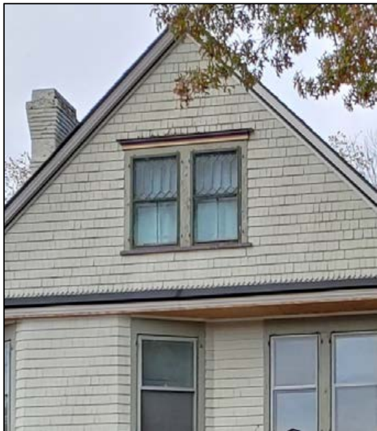
Original windows left intact and maintained.
