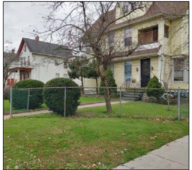
Inappropriate chain link fence.
