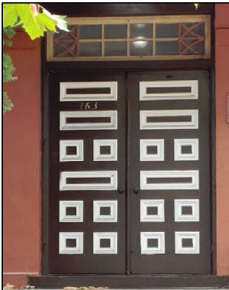
Original wood door and transom.
