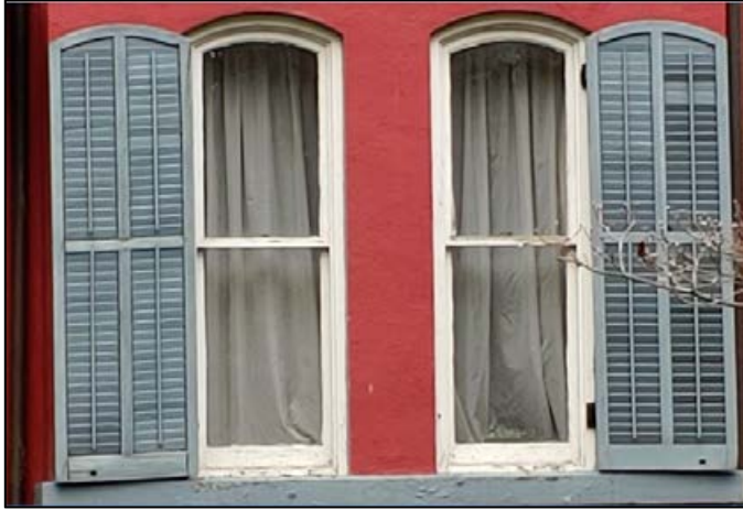
Original stucco, wooden windows, and appropriate shutters.
