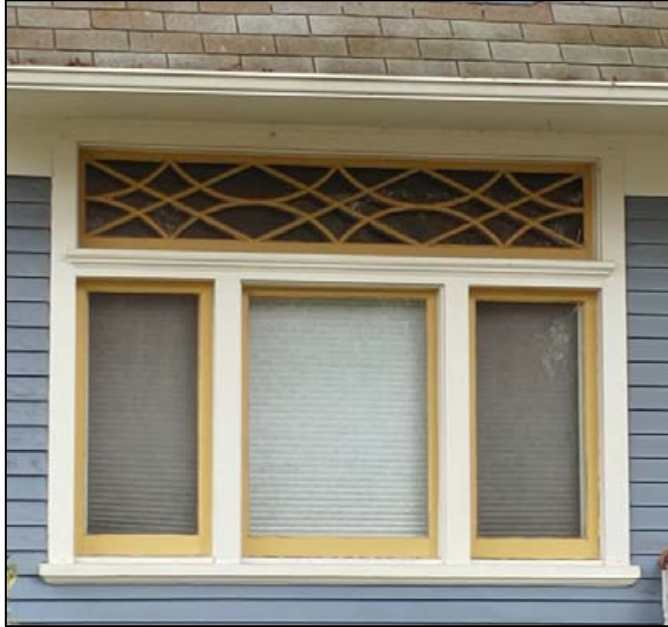
Well-maintained original wood single hung and leaded transom windows.
