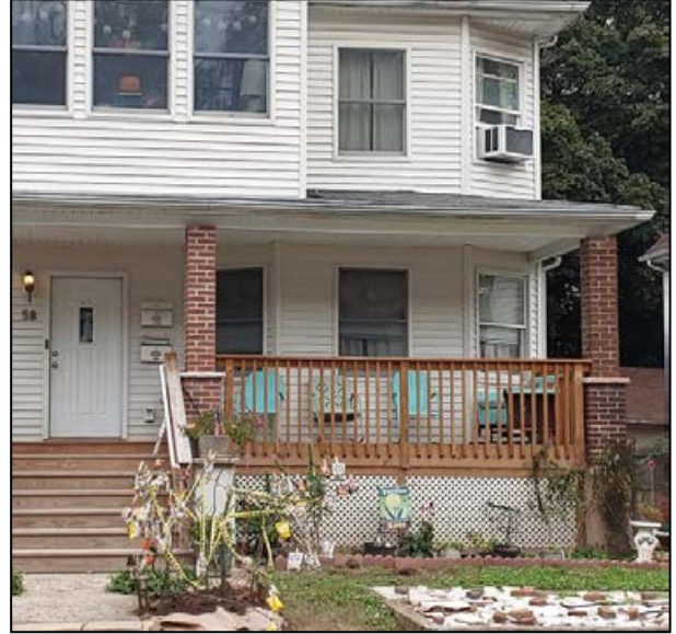
Air conditioning unit on the front elevation.
