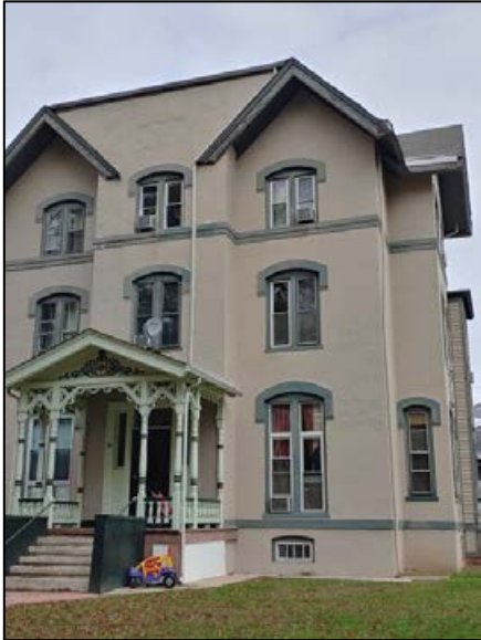
Satellite dish installed on side entry.
