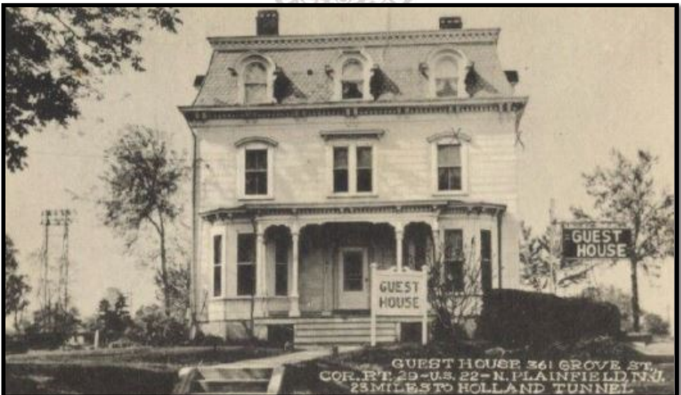
Figure 25 Historic View of Residence at 361 Grove Street.
